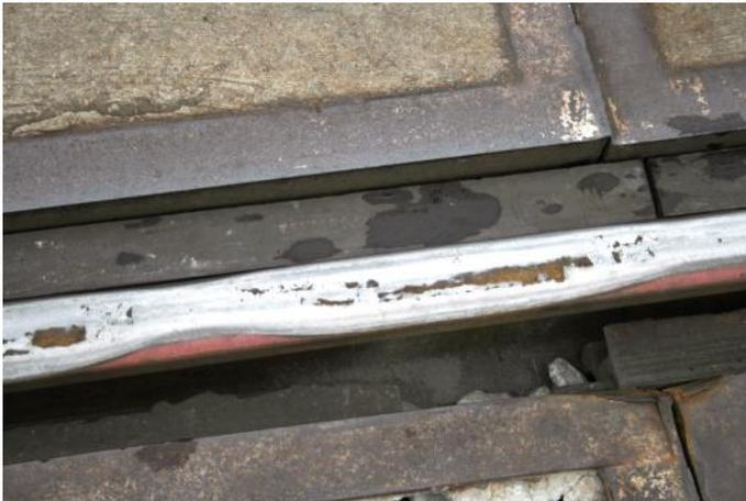
The wear on the railhead is particularly acute on curves, and rail grinding trains might need multiple passes to get the railhead ground to just the right profile given the degree of curve, train speeds, and train weight. This calls for careful analysis of the rail line, and careful control over the grinding mechanisms. The host railroad and the rail grinding experts arrive at detailed grinding plans before work commences.
