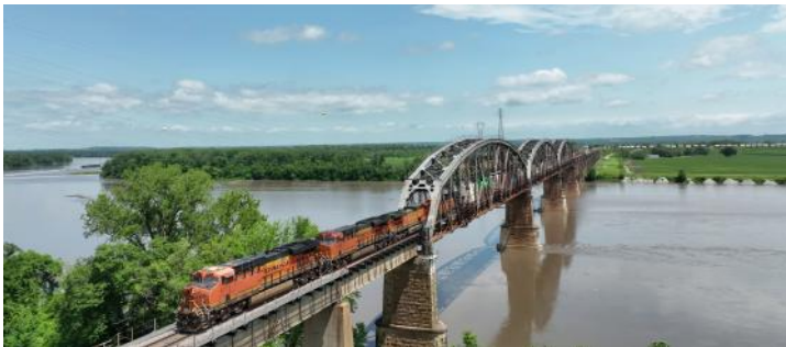
BNSF bridge at Sibley MO June 2025
