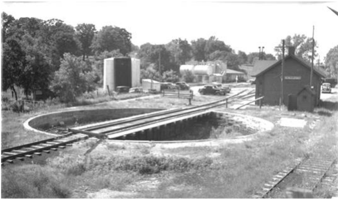
C&NW turntable and depot at Benton, Wisc, 1947. Photo by F. R. Ritzman, collection of LSRHA.
