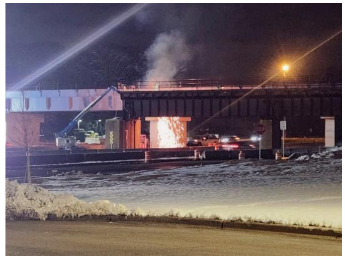
The old bridge being removed on January 11, 2024. Photo by Dave Rasmussen.
